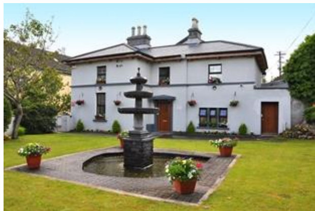
Pictured above: Canal House, Ballinasloe, Co. Galway.
